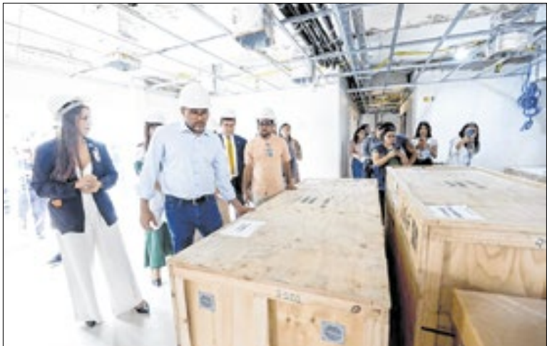
Wilson Lima vistoriou as obras do Hospital-Dia
