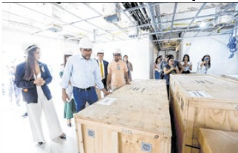
Wilson Lima vistoriou as obras do Hospital-Dia
